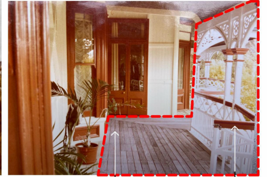
VERANDAH RAIL DETAIL FLOOR/SQUARE BOARD DETAIL
