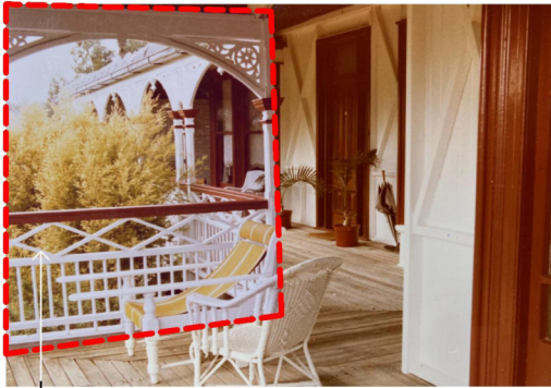
BALUSTRADE AND VERANDAH BEAM DETAIL POST DETAIL AND SURROUNDS BALUSTRADE TOP, BOTTOM AND MID-RAIL DETAIL
