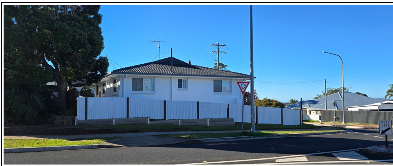
PHOTOGRAPH 2 - View of the site from Rowbotham Street.
