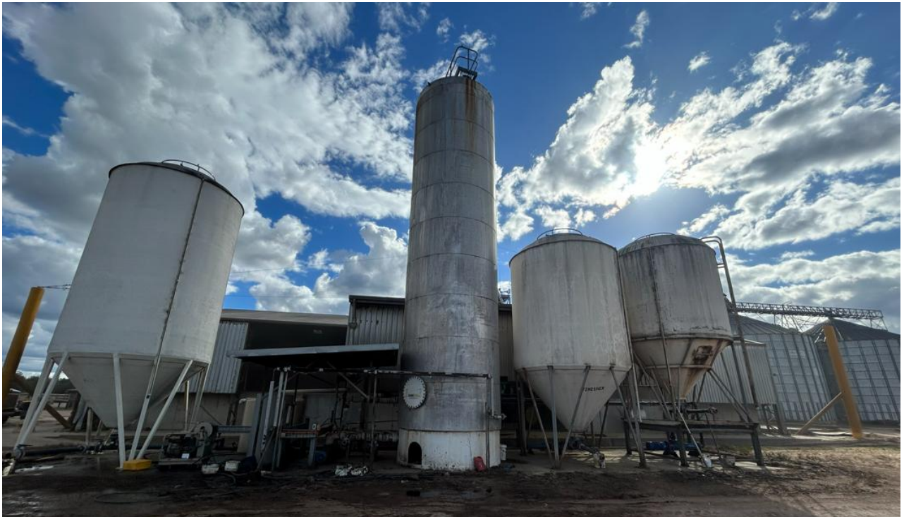
Figure 22. Liquid additive tanks.
