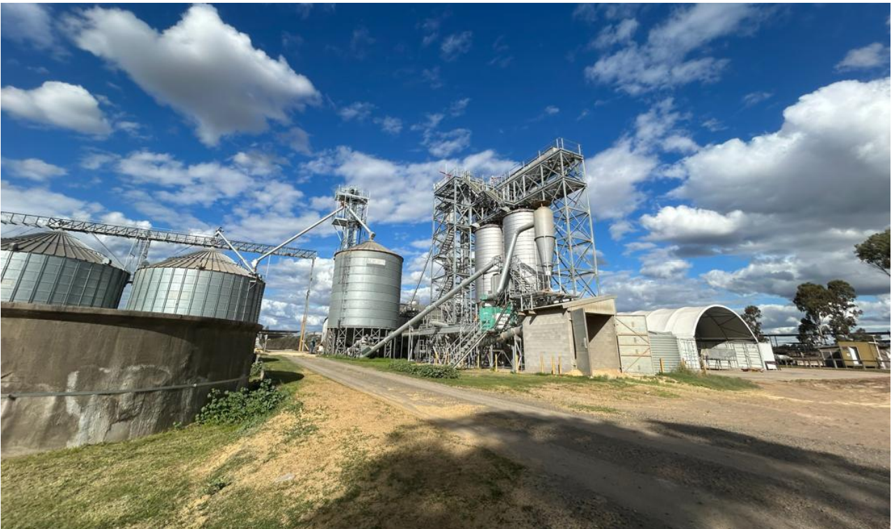
Figure 19. Grain delivery road and mill structure.
