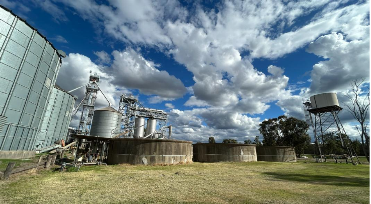
Figure 20. Grain and water storage.
