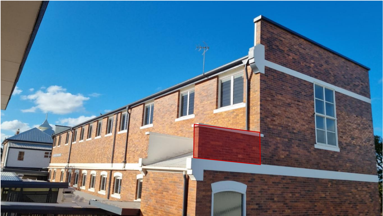
Figure 12 Detailed view of the single storey wing, rear of the Archbishop Dunne Building, with the section of the parapet wall to be demolished highlighted in red Source: Aspect APM, annotated by Lovell Chen
