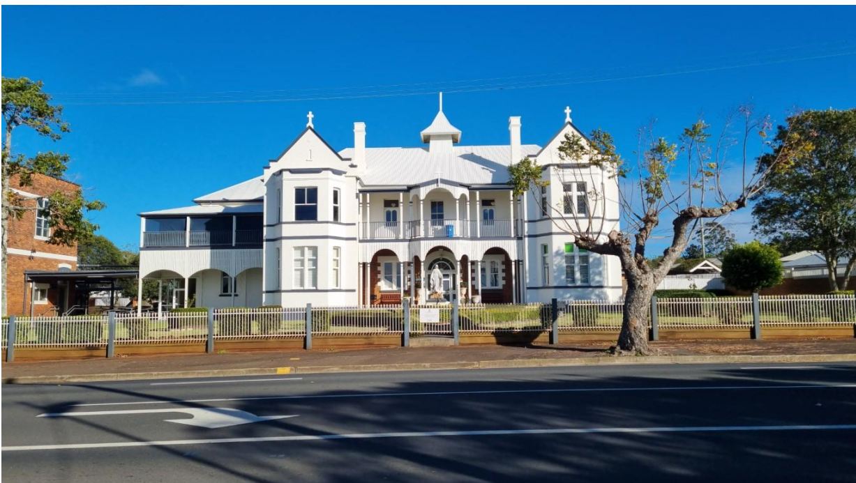
Figure 9 Front (east) elevation of Brothers' House along West Street Source: Aspect APM
