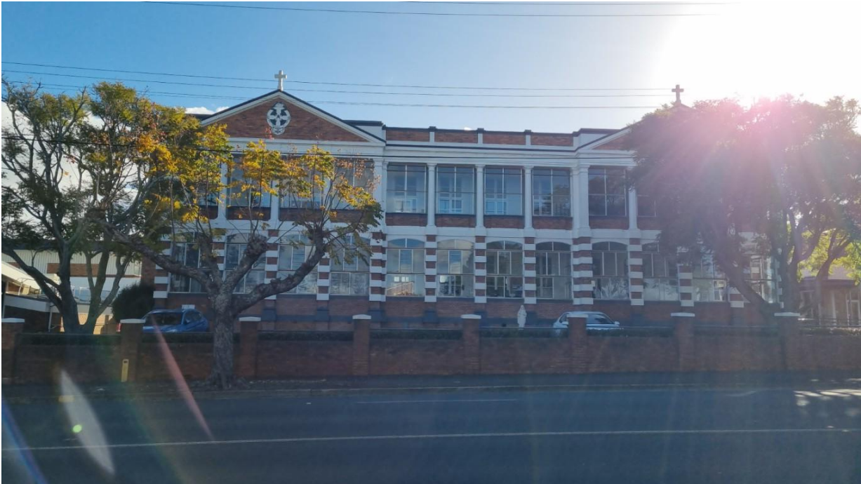
Figure 10 Front (east) elevation of Archbishop Dunne Building along West Street. Note the verandahs are enclosed with modern glazing Source: Aspect APM
