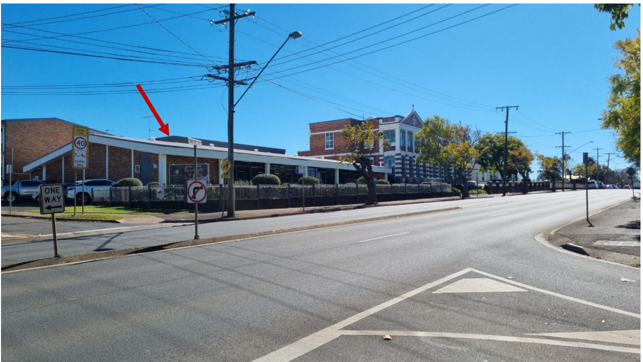
Figure 7 View of the St Mary's College campus from the intersection of West and Hill streets. Note the single storey T P O'Brien building proposed for demolition indicated by the red arrow Source: Aspect APM
