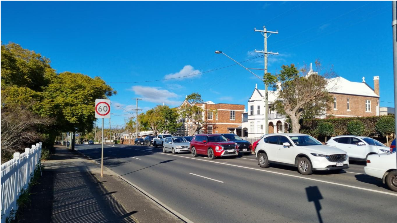
Figure 8 View of the Brother's House and Archbishop Dunne Building along West Street, facing south Source: Aspect APM
