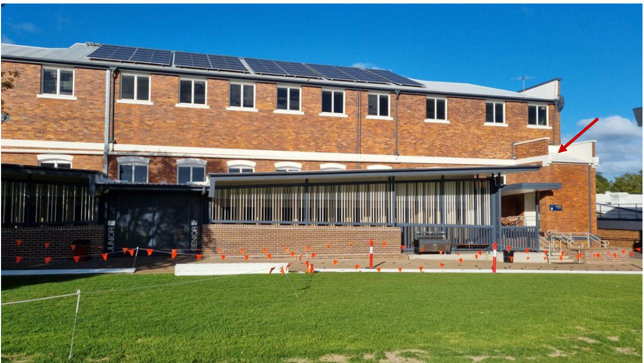
Figure 11 Rear (west) elevation of Brothers' House showing the single storey wing and the proposed location of the new skybridge indicated Source: Aspect APM
