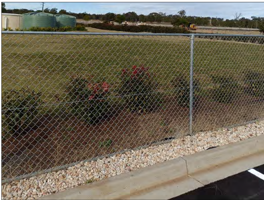
Plate 2: Chain link Mesh fence installed around the internal site.
