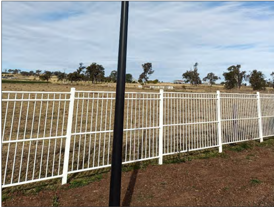
Plate 1: Aluminium fence currently installed along the eastern boundary of the site
