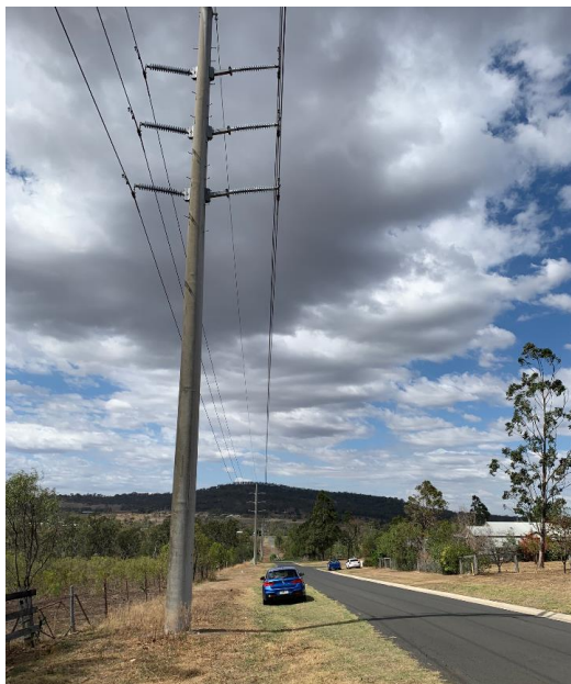
Figure 1: Northern Boundary St pole
