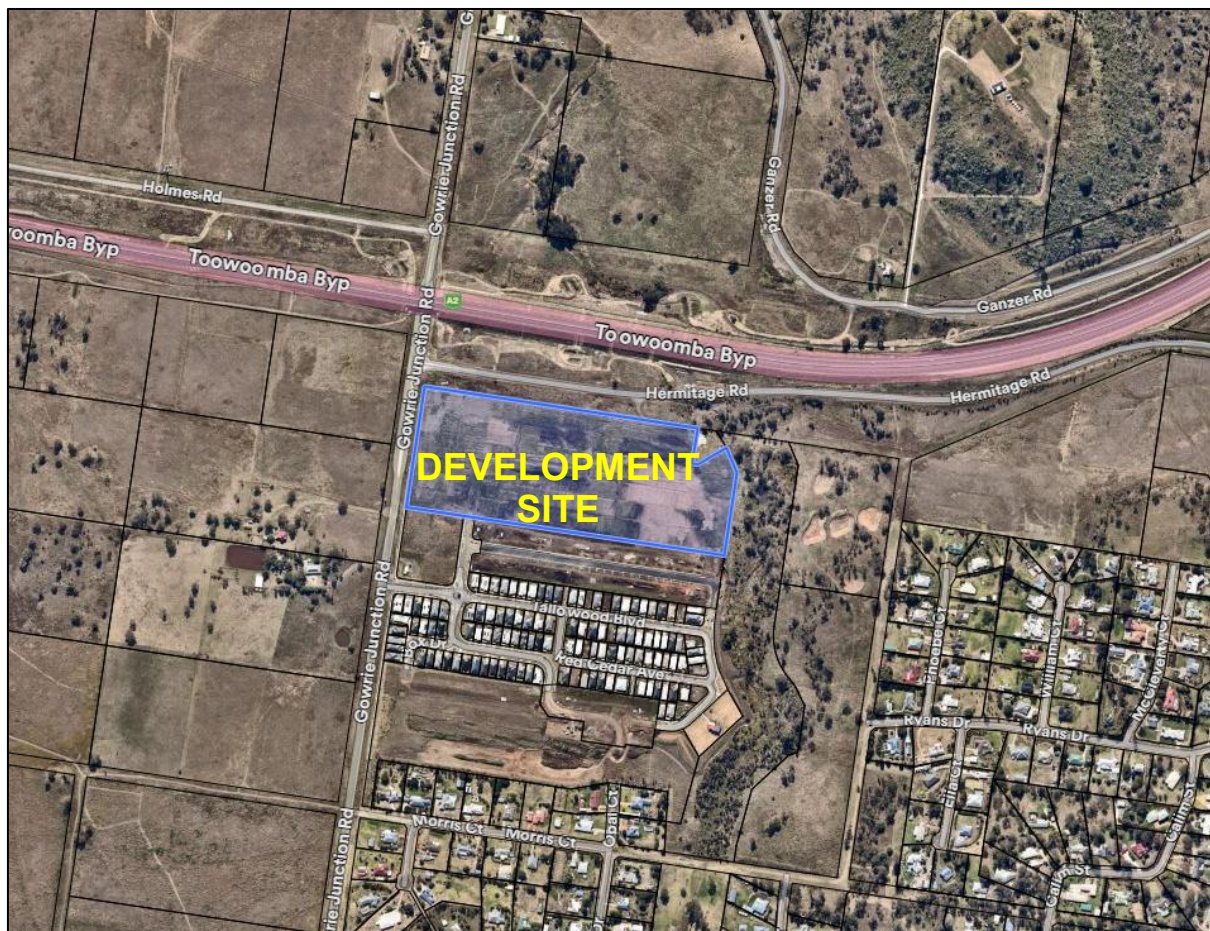
Figure 1 – Indicative site location (Nearmap, 2024)
