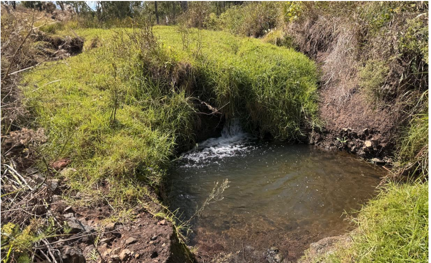
Figure 5 Photos illustrating existing eroded condition of waterway within subject lot
