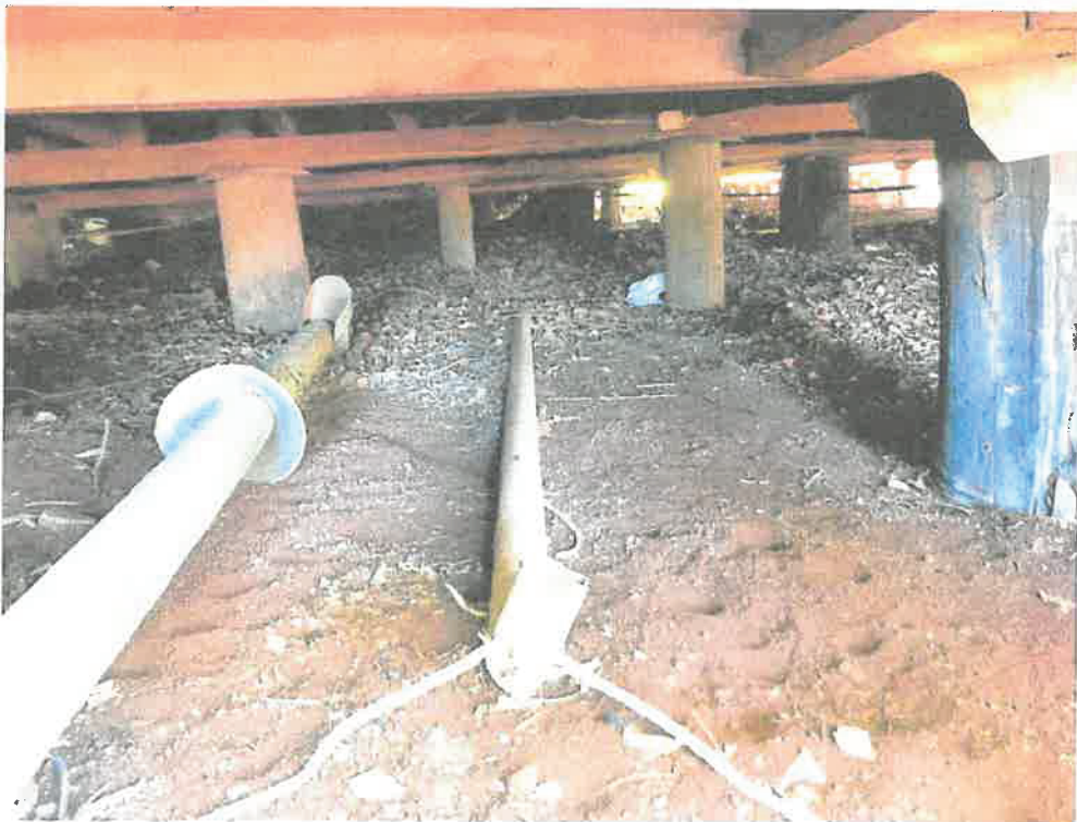
Photo 2 – View of Underfloor
