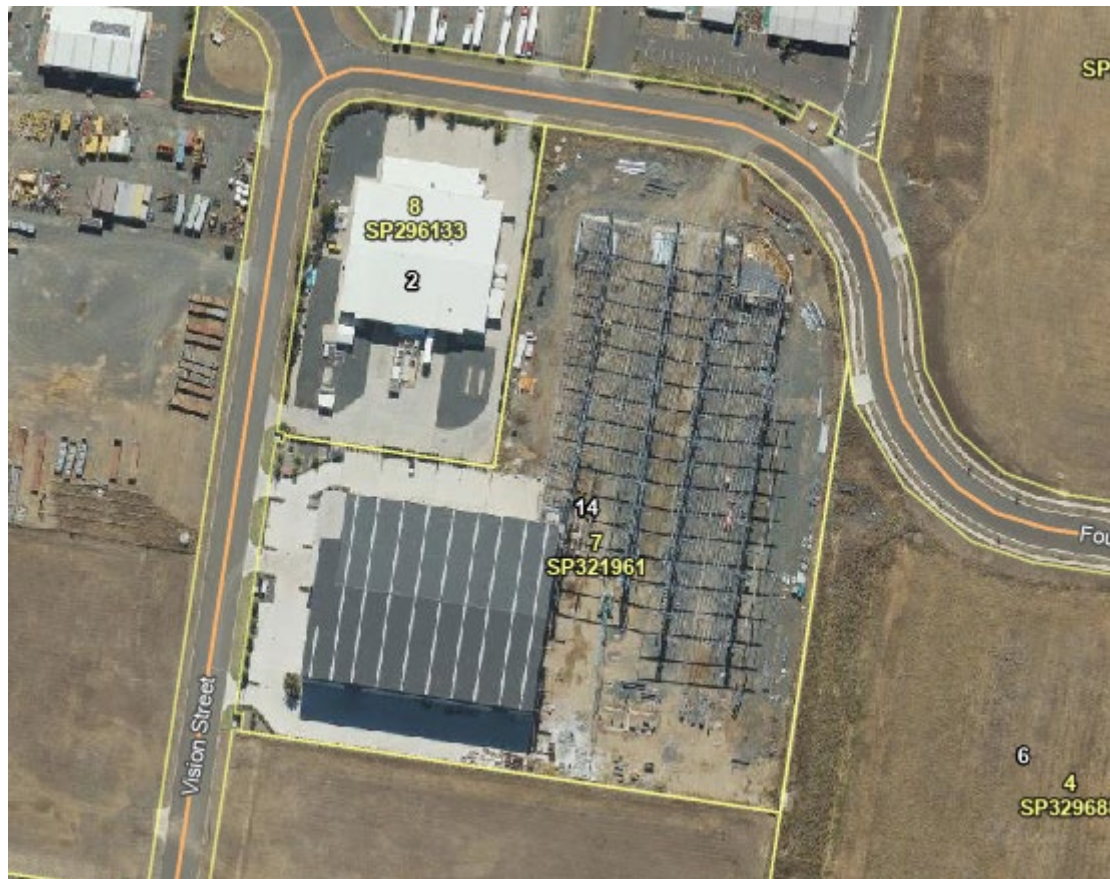
Extract 1 – Subject Site Source – Queensland Globe
