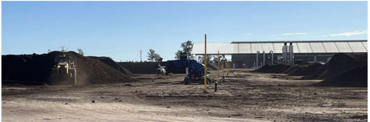
Fig 3 - Windrows and hydrants on composting pad
