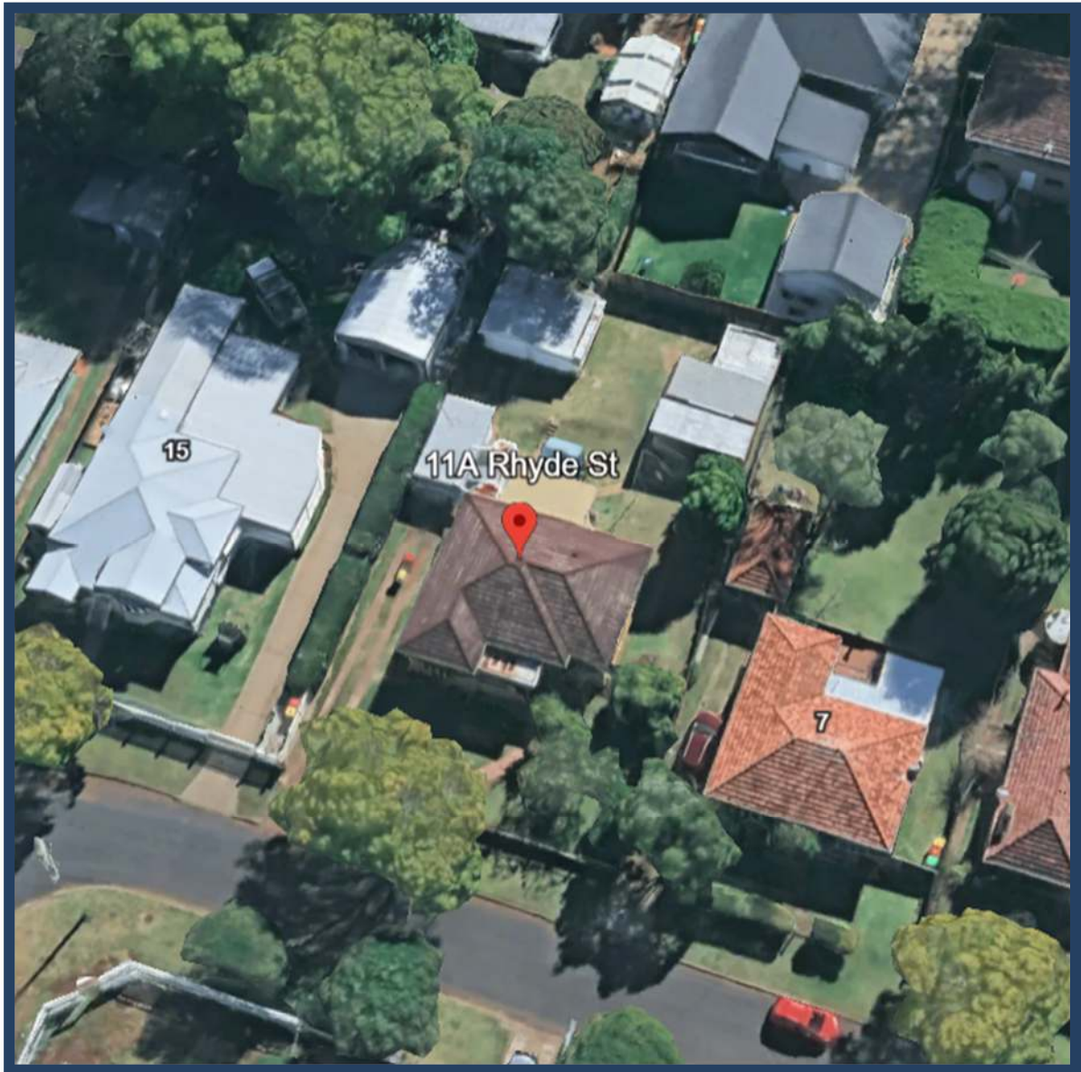
Figure 12: Aerial view of existing dwelling house use
