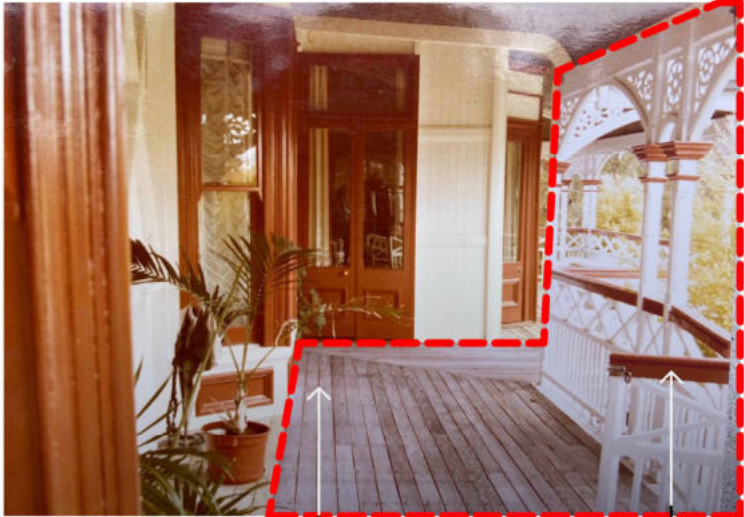
VERANDAH RAIL DETAIL FLOOR/SQUARE BOARD DETAIL
