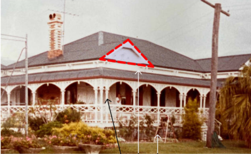
INFILL UNDER BALCONY CHIMNEY CAP DETAIL VERANDAH BALUSTRADE POST DETAIL GABLE FRETWORK AND FINISH DETAIL
