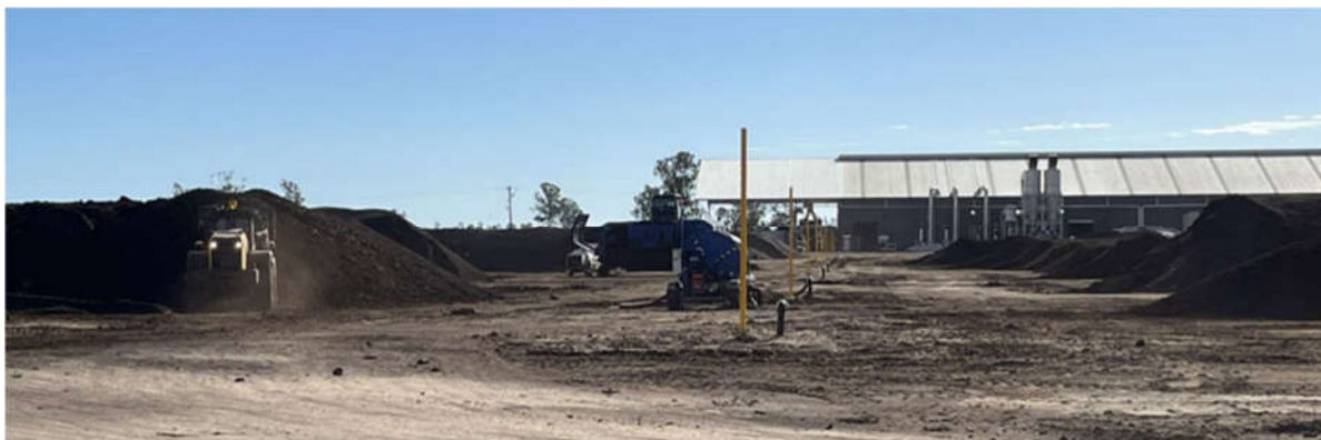
Fig 3 - Windrows and hydrants on composting pad
