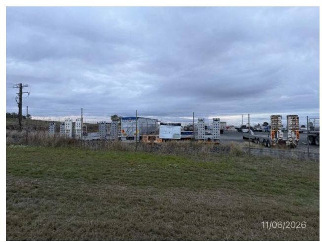
FIGURE 6 – Sign on Wirths Road Frontage - Location
