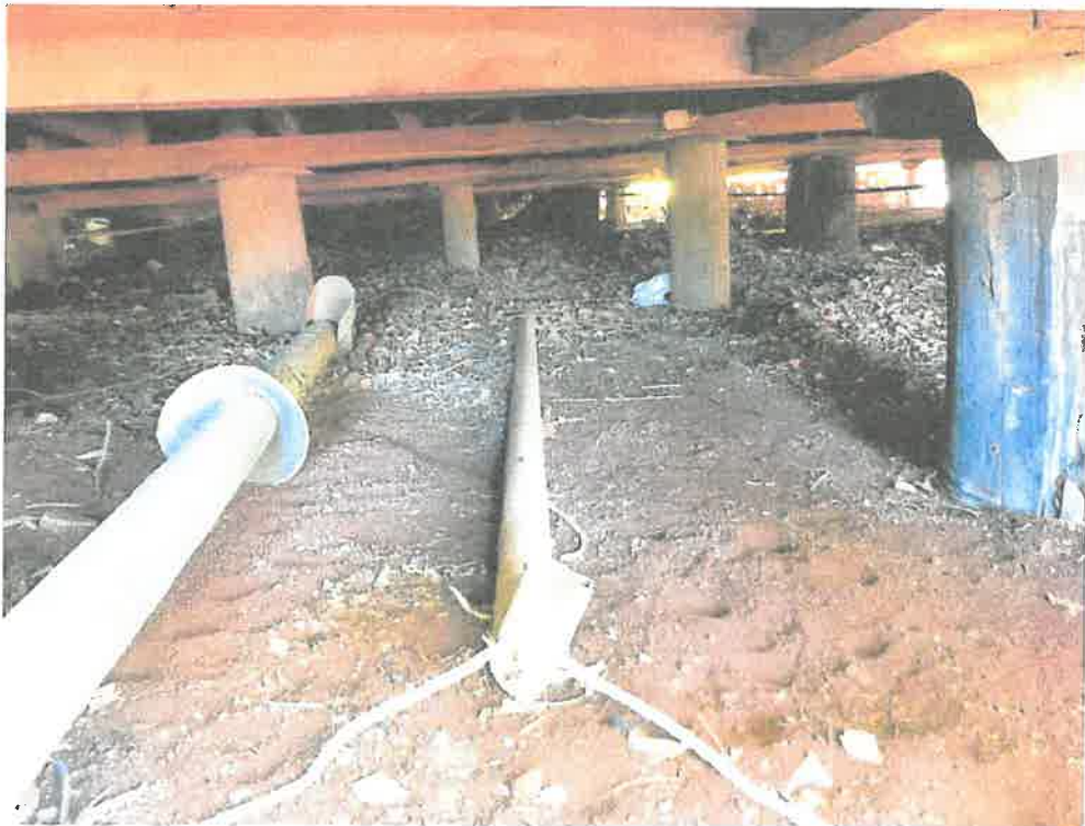
Photo 2 – View of Underfloor
