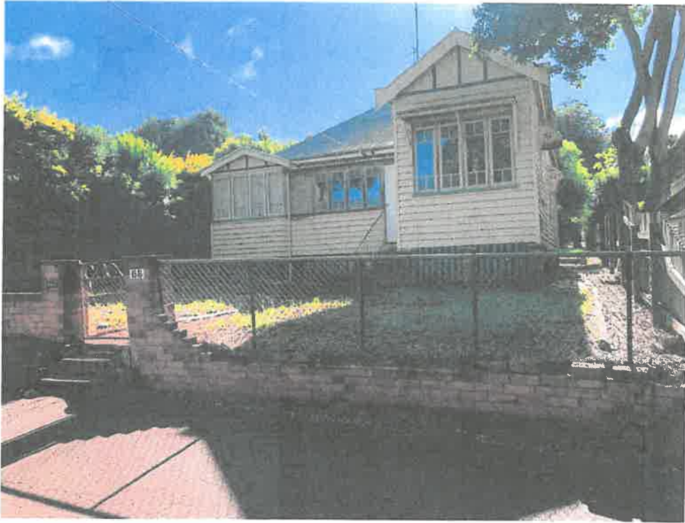
Photo 1 – View from Hume Street of the Residence.
