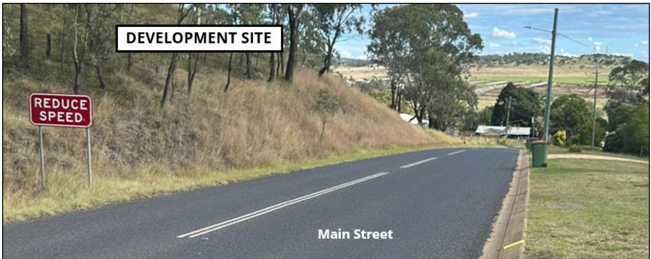
Figure 2-3 Main Street Facing West at the Site's Frontage (Source: Site Visit, 2025)
