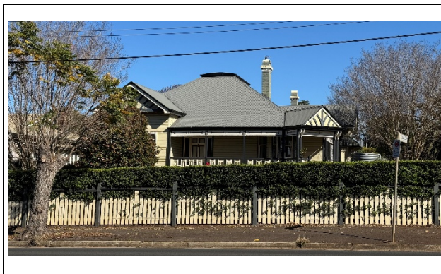
PHOTOGRAPH 8 - Front view of the residence at 133 West Street to the south of the development site area taken from the West Street frontage.
