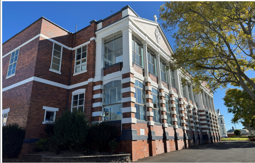
PHOTOGRAPH 3 - Front view of the Archbishop Dunne Primary Building to the north of the development site area.
