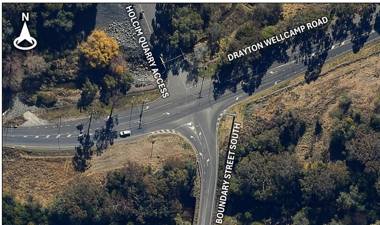
Figure 3-4: Drayton Wellcamp Road / Boundary Street South / Holcim Quarry Access
