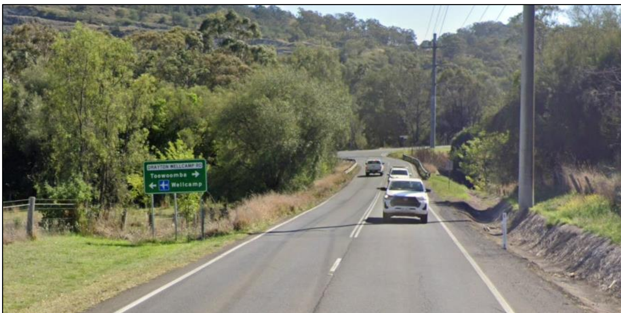
Figure 3-2 Boundary Street South looking north towards Drayton Wellcamp Road
