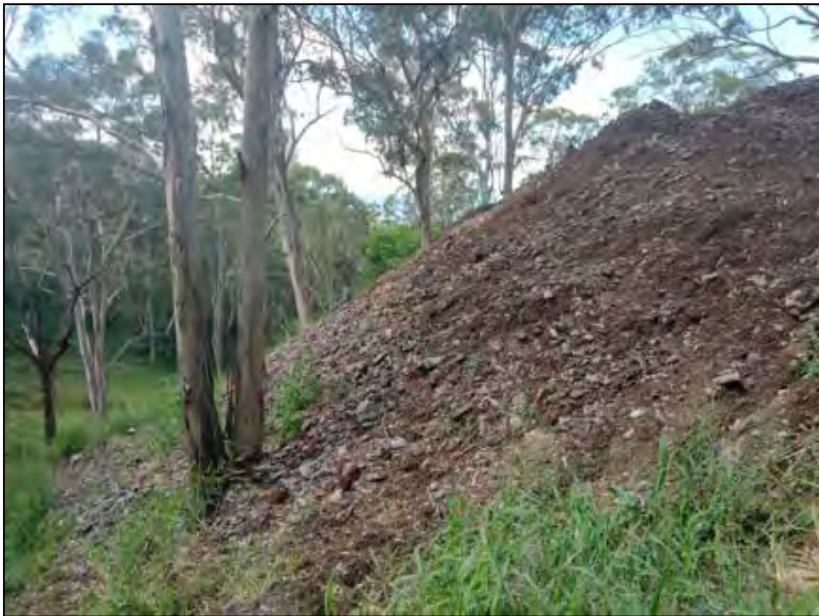
PLATE 5 – CLOSE UP OF FILL BATTER
