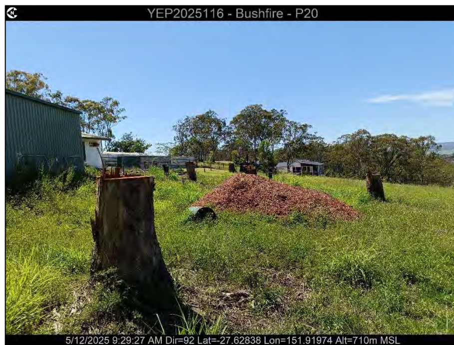
Plate 6: Chopped down and mulched trees on site
