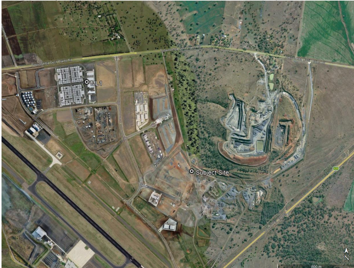
Plate 3.1: Showing the approximate noise measurement location (ML1) in relation to the subject site.
