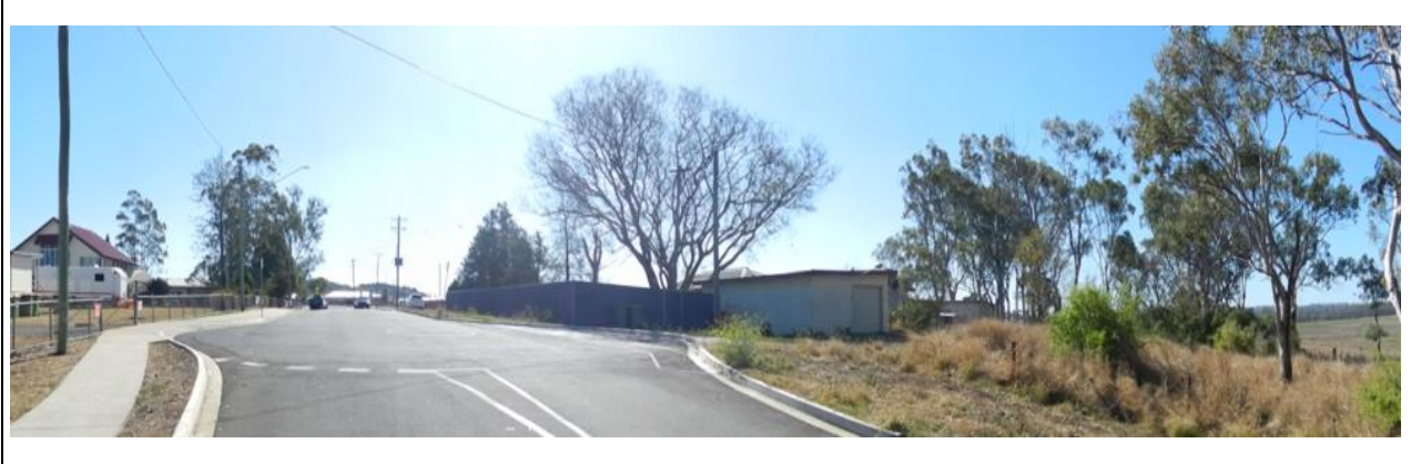
PHOTOGRAPH 5 - View looking west along Meringandan School Road towards the existing dwelling and associated outbuildings that will be demolished and removed as part of the establishment of an approved Child Care Centre.
