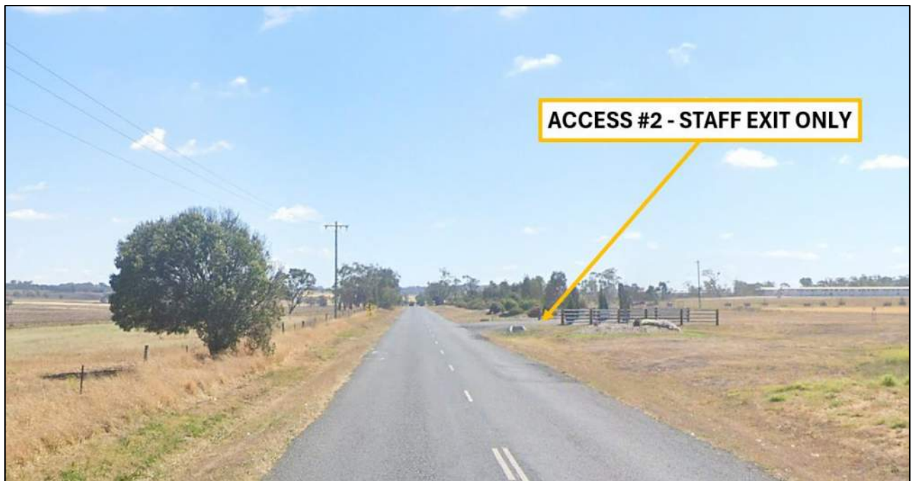
Figure 3-2: Clifton Road (looking north)
