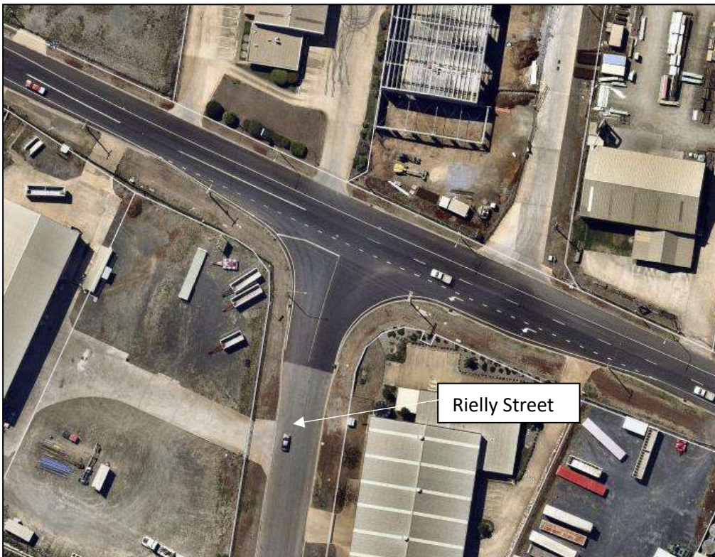
Carrington Road / Rielly Street intersection
