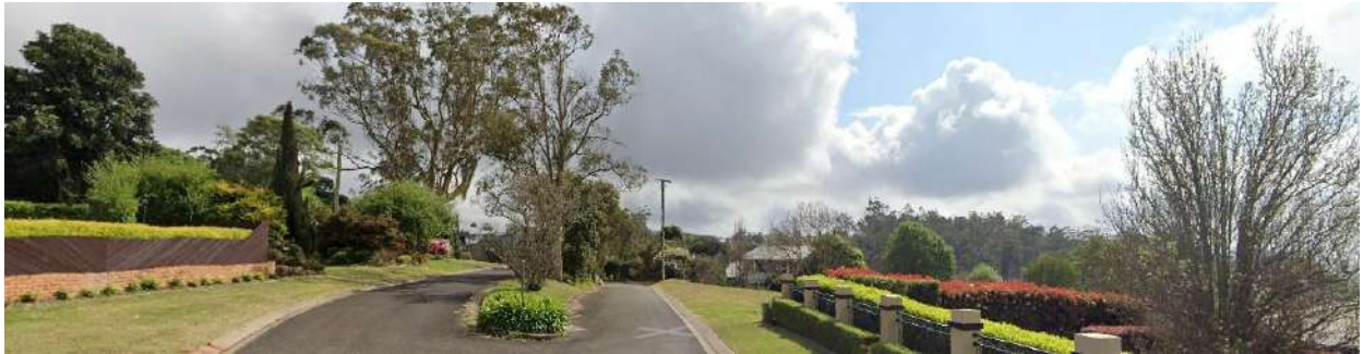
Photos 2: Three images of a street (Culliford Drive) that has been split to ameliorate differential levels in its cross-section
