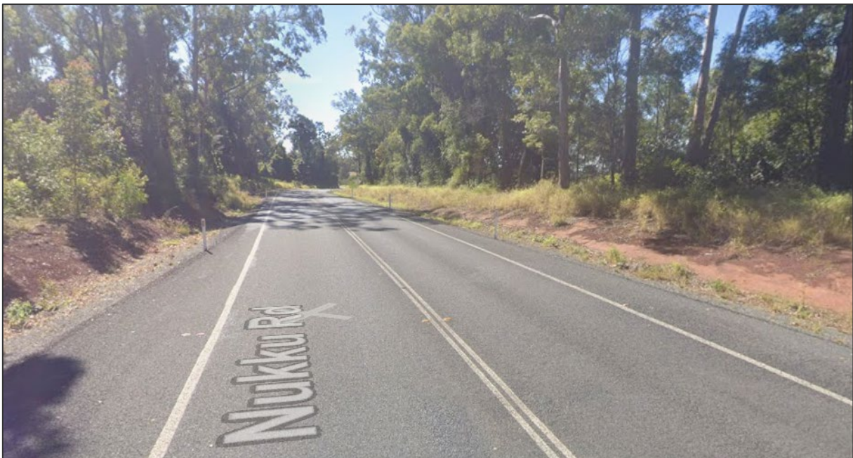
Figure 4: Nukku Road north of the Ness Wilson Road intersection (Google Street View, 2026)
