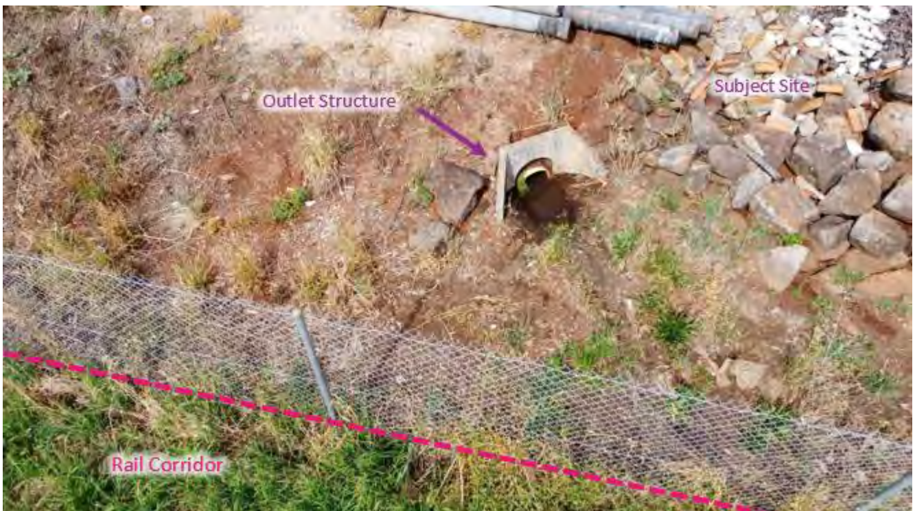
Figure 3-6 Railway Corridor Outlet Structure
