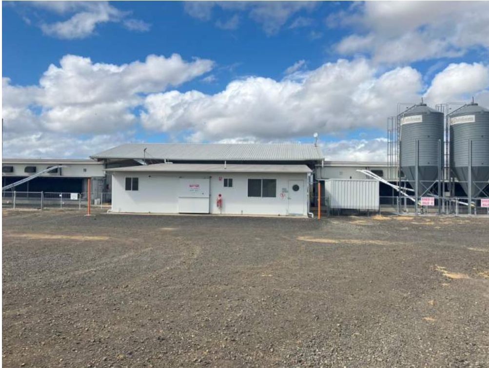
Photograph 5 – Central amenities building shared by a pair of sheds
