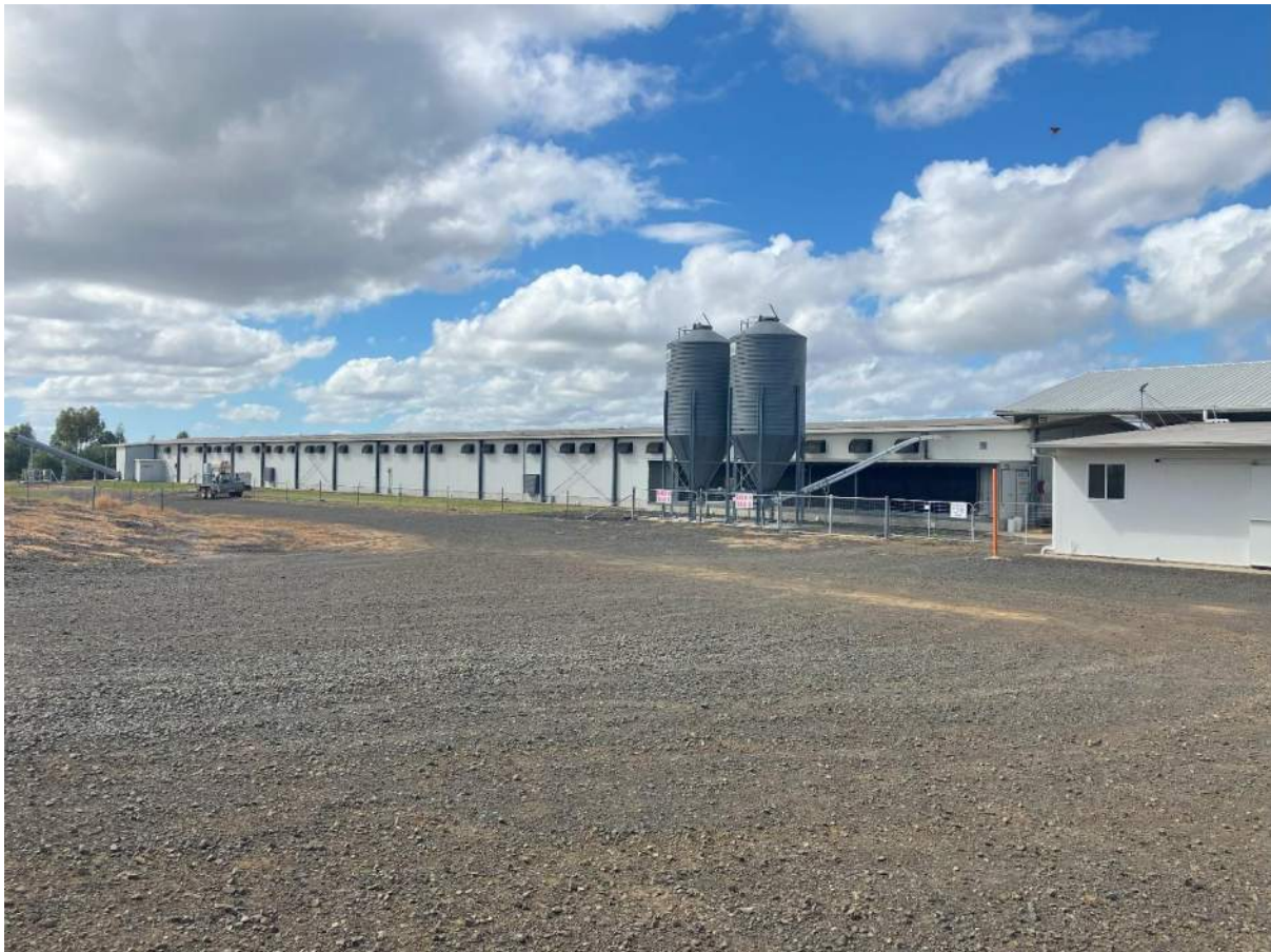
Photograph 1 – Single shed with ancillary infrastructure
