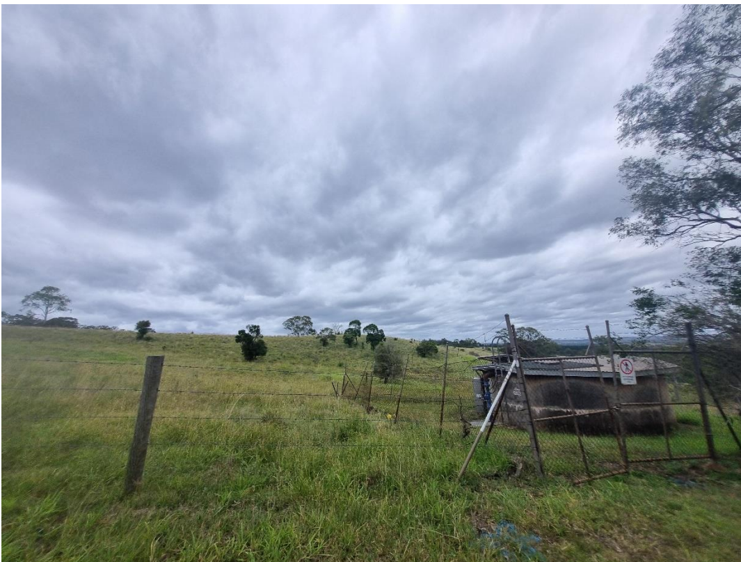
Photograph 2 View looking west of the existing reservoir to be decommissioned (Lot 3 RP117988).
