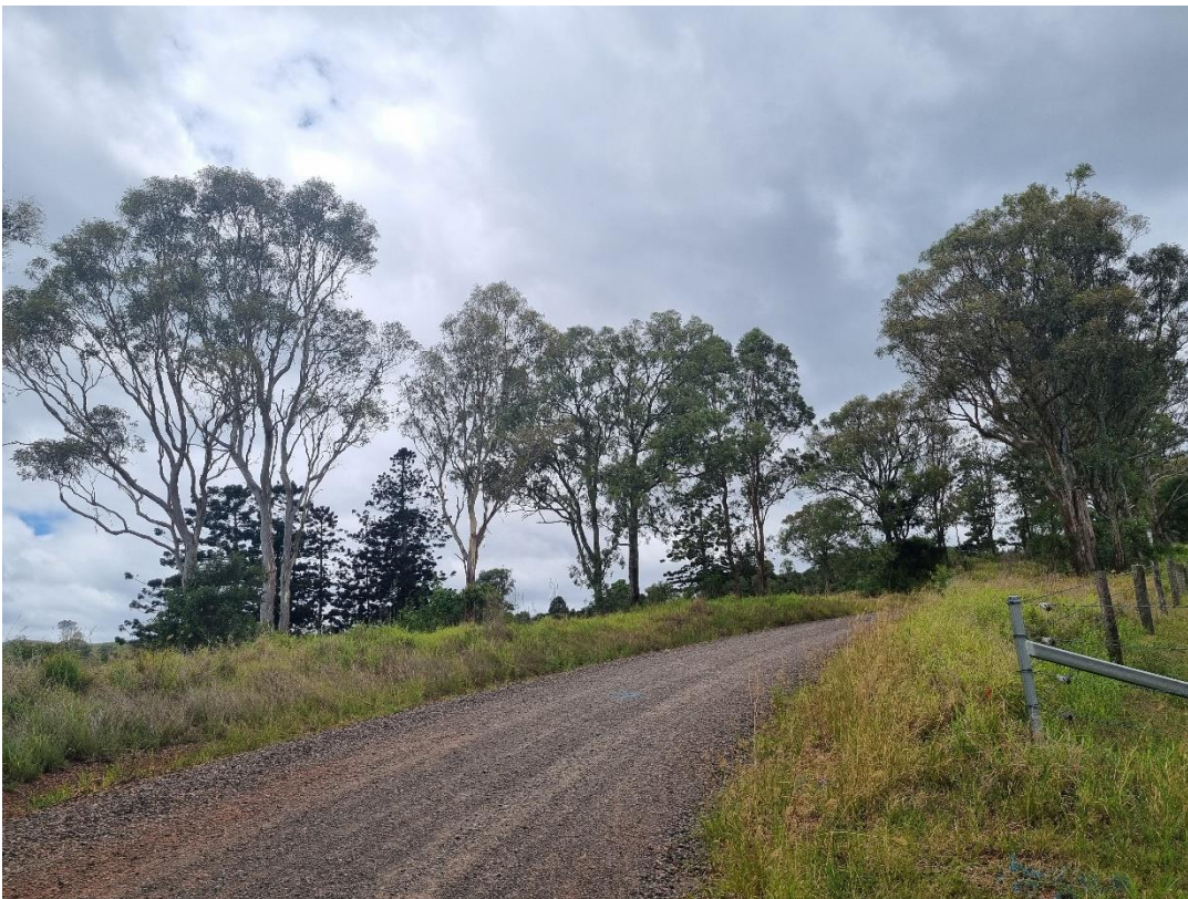
Photograph 4 View looking south from the approximate end location of the pipeline replacement works (-27.3009, 152.0730).
