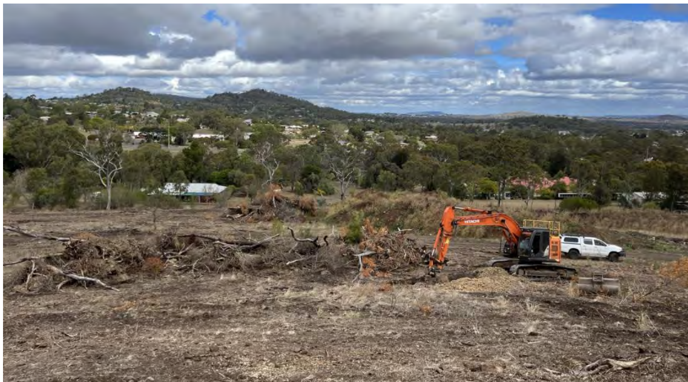
Image 7: General site conditions looking south toward TP8
